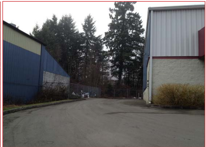
Generous sized access to the rear of the building
