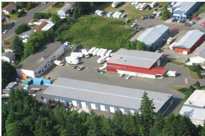
Aerial view of the property
